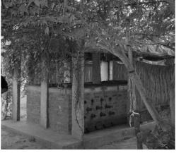
Fig. 1. Box composting by the RISE Citizens Initiative in Bangalore. The compost boxes, covered by a roof structure, are brick built with passive aeration vents and a lockable metal grille cover to hinder indiscriminate dumping by residents and to prevent rodents and vectors from entering the compost pile.
